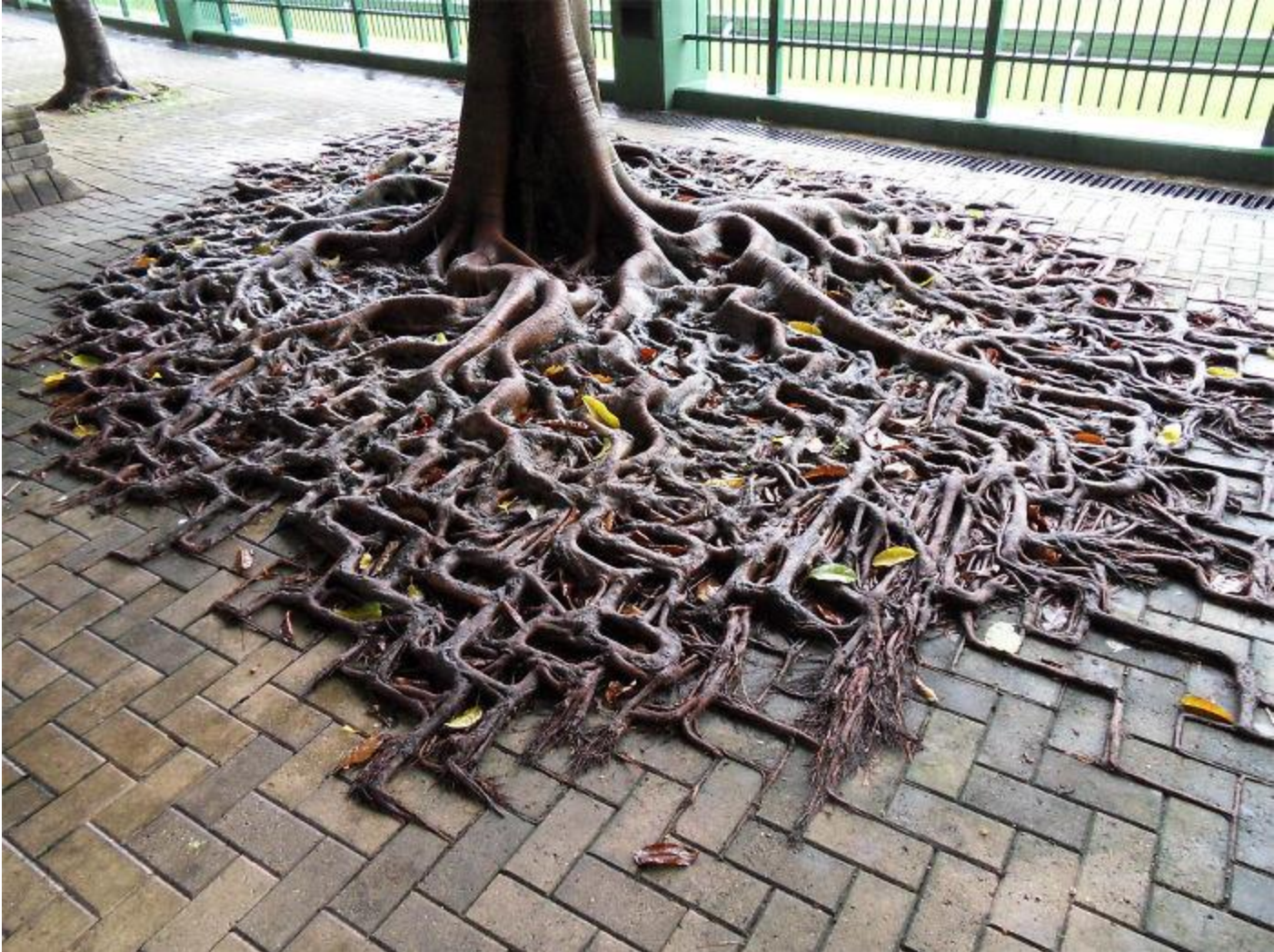
A Tree's Roots That Spill All Over The Sidewalk
